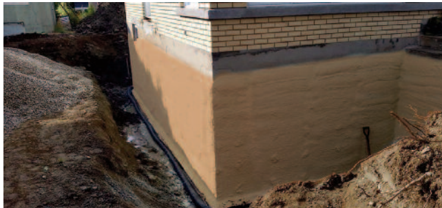
When an old foundation is excavated, it is the ideal time to insulate them by the exterior with spray polyurethane foam.
