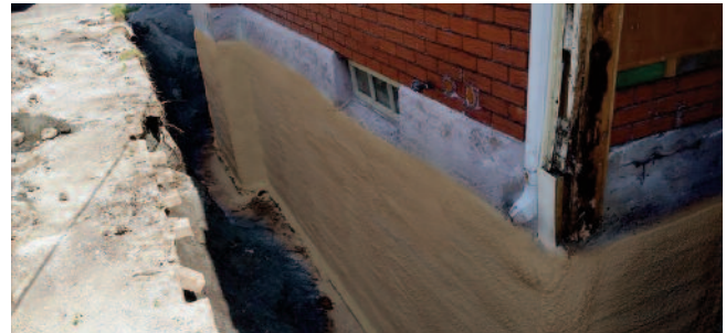
When an old foundation is excavated, it is the ideal time to insulate them by the exterior with spray polyurethane foam.
