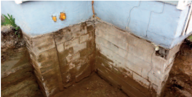
Foundation before being repaired
